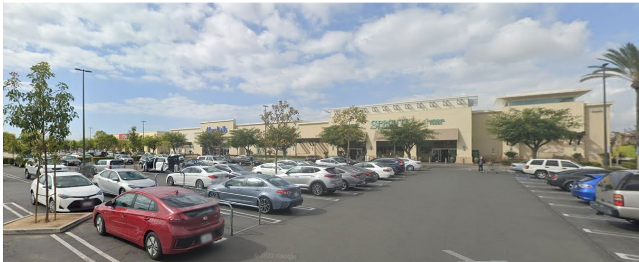
Photograph 4. View of Buildings 4A–4C, looking southwest (Google Street View, March 2021).
