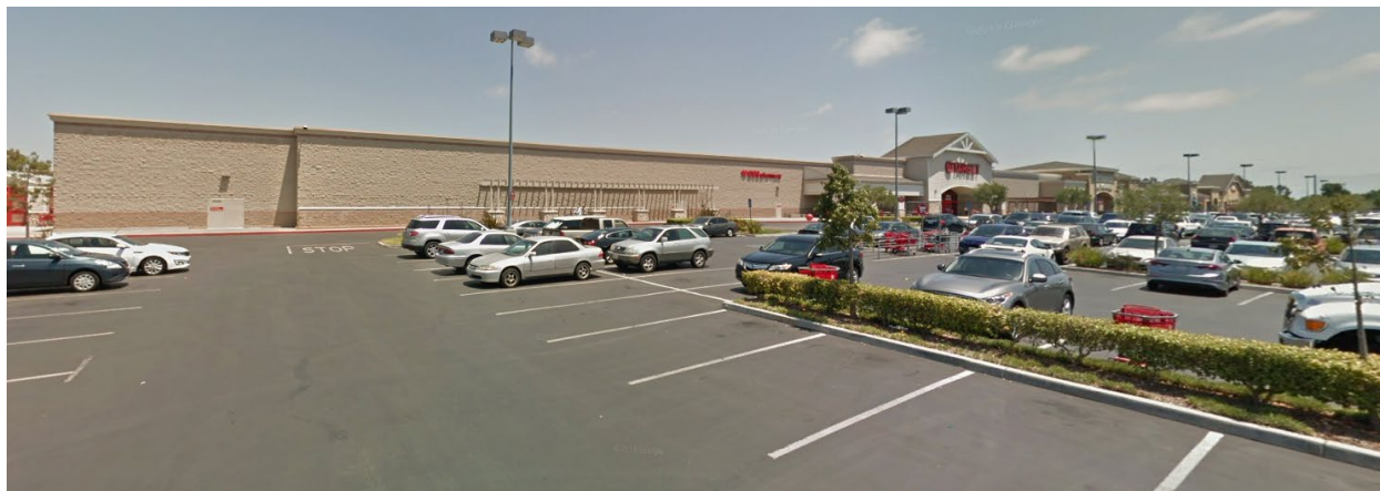
Photograph 7. View of Building 5A and 5B, looking southeast (Google Street View, June 2017).
