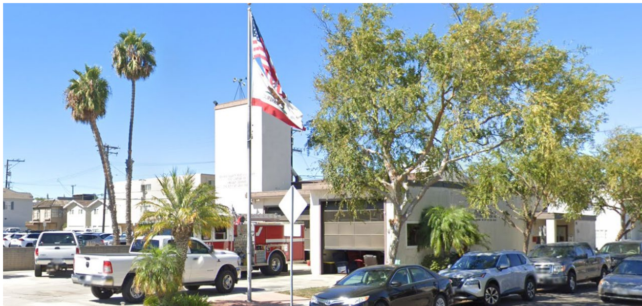
Photograph 17. View of the Orange County Fire Station 44, looking southwest (Google Street View, September 2022).
