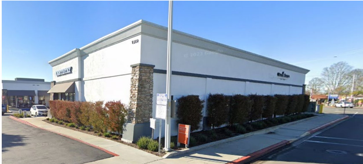
Photograph 10. View of Building 6B, looking southwest (Google Street View, January 2023).
