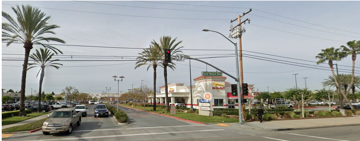
Photograph 6. View of Building 5H, looking northwest (Google Street View, January 2023).
