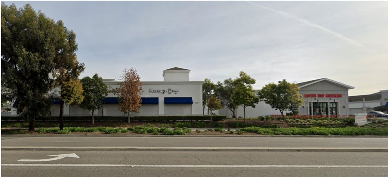
Photograph 8. View of Building 5G and 5H, looking east (Google Street View, January 2023).
