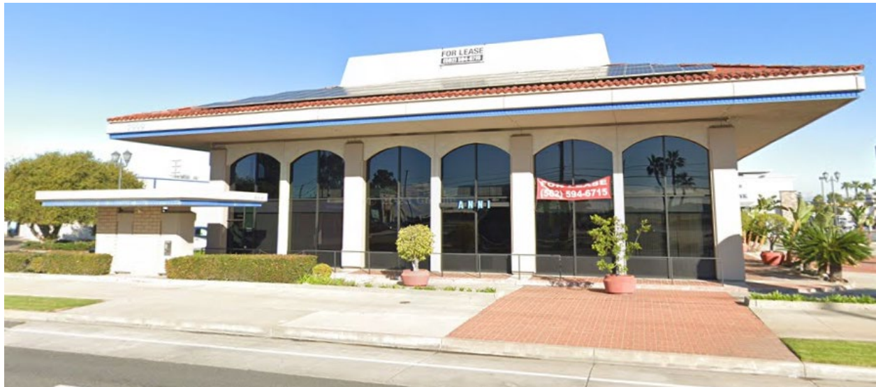
Photograph 13. View of Building 6L, looking northwest (Google Street View, January 2023).
