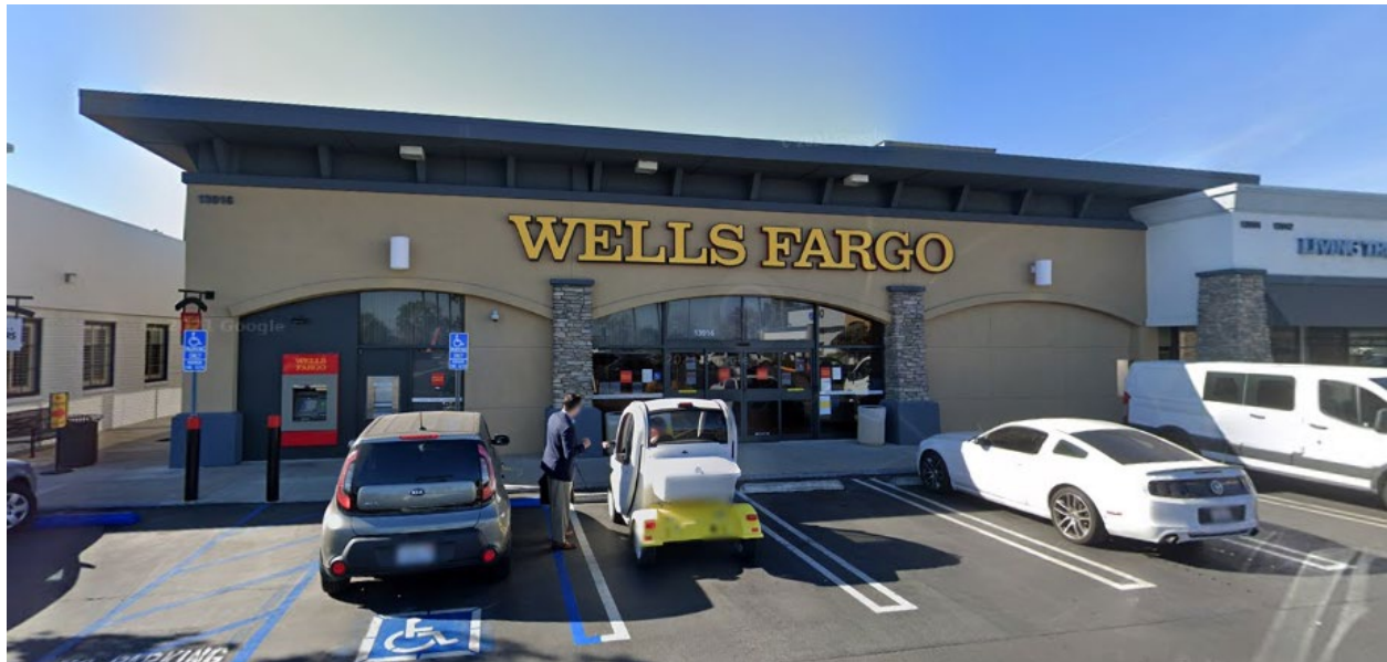
Photograph 11. View of Building 6D, looking west (Google Street View, January 2021).
