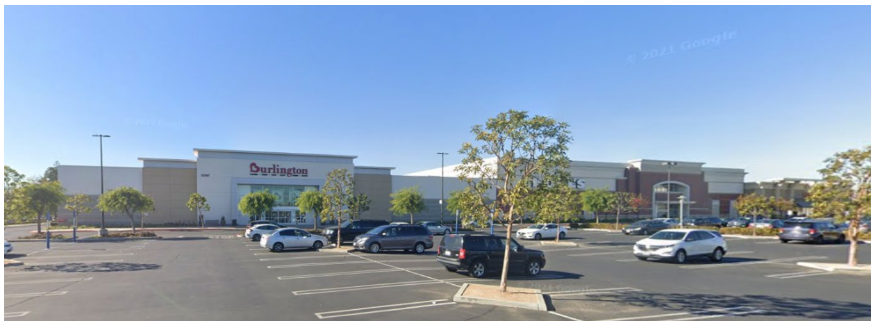
Photograph 5. View of Buildings 4E and 4F, looking northwest (Google Street View, January 2021).
