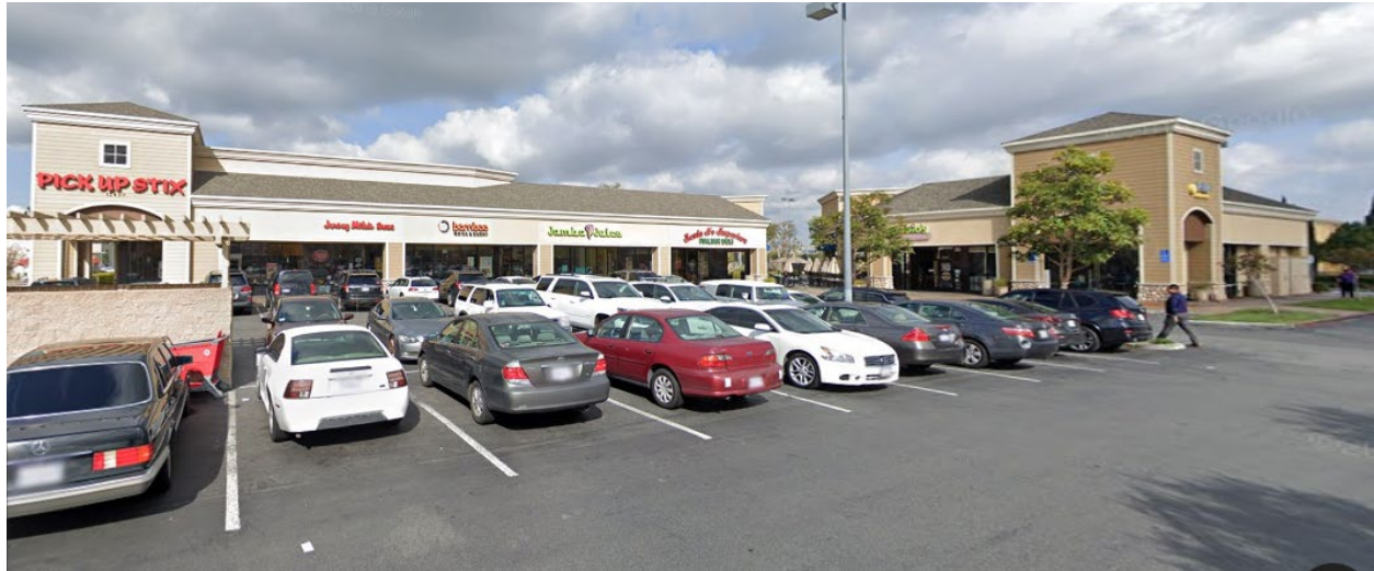
Photograph 9. View of Building 5I and 5J, looking northwest (Google Street View, March 2019).
