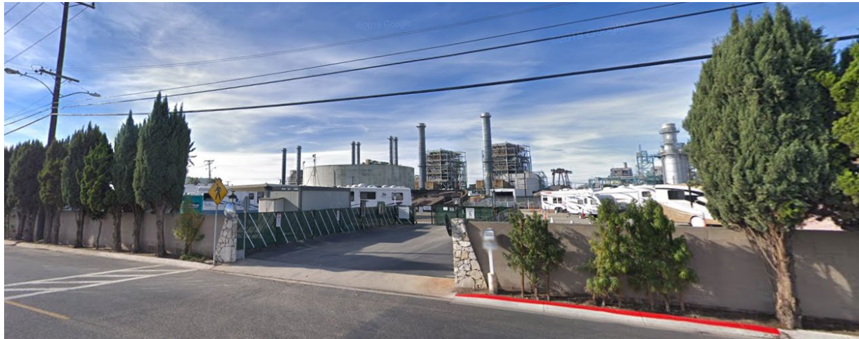
Photograph 2. View of Site 2, looking southwest (Google Street View, January 2018).
