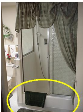
Before Cut Down
