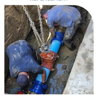
Staff replaced a 6" water main line valve located in Leisure World that has reached the end of its serviceable life. Main line valves enable staff to isolate smaller portions of the water system during maintenance and repairs resulting in less customers affected by necessary shutdowns.
