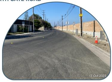
As part of the I-405 Widening Project restoration efforts, an access driveway that leads to the City's Beverly Manor Reservoir was replaced. This driveway also provides access to telecommunication providers, Caltrans, and numerous utility companies. Additionally, OC405 restored a 700-foot-long section of asphalt along North Gate Road.
