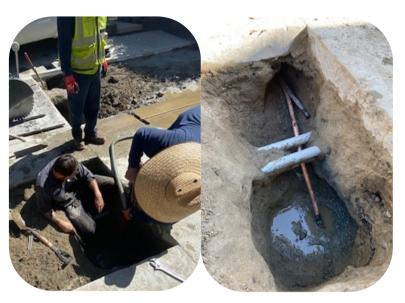
While performing a maintenance request, staff discovered a residential water service line in Old Town made of plastic polybutylene. Polybutylene becomes rigid and brittle over time making it a difficult material to work with. Staff excavated the existing service line and replaced it with a new 1" copper line.
